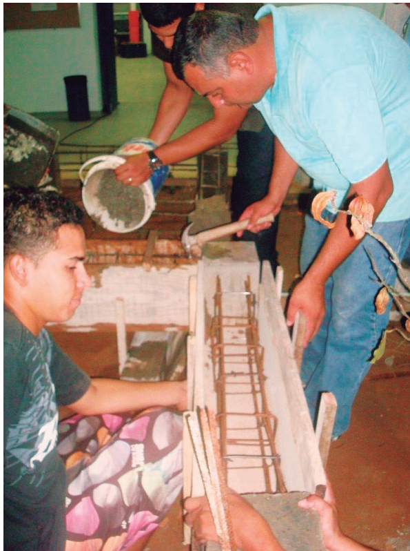
Figure 3 - The students building the structures – Phase 3: throwing and modelling the concrete
