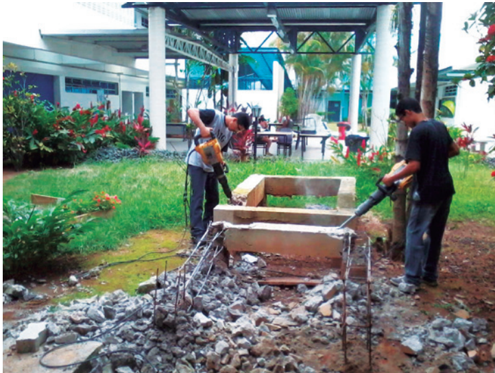
Figure 4 - The students deconstructing the structures
