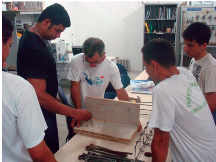
Figure 1 - The students building the structures – Phase 1: shaping wooden formwork for reinforced concrete
